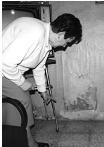
Tenant points to a deteriorating wall
